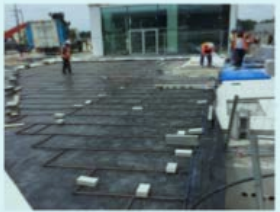
Installation of the injection network and evaporative pavements
